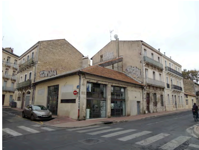
Restructuration de hangar
